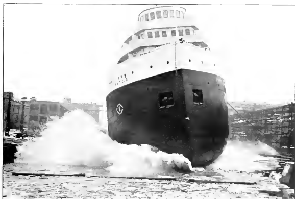
An interesting view showing the sidewise launching of the William K. Field, 12,000 deadweight ton bulk freighter for Great Lakes service built at the yard of the Toledo Shipbuilding Company, Toledo, Ohio; launched January 24, 1924.
